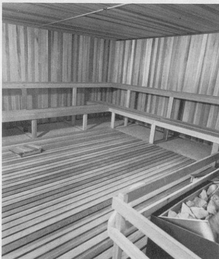
Yes, it's true—the McClain Facility even boasts a sauna and steam room.
