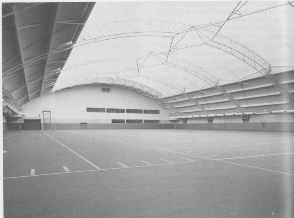
The focus of the McClain Facility is, of course, the 90-yard artificial turf practice field. The 76,380-square-foot main floor even has enough height for kicking and punting practice.
